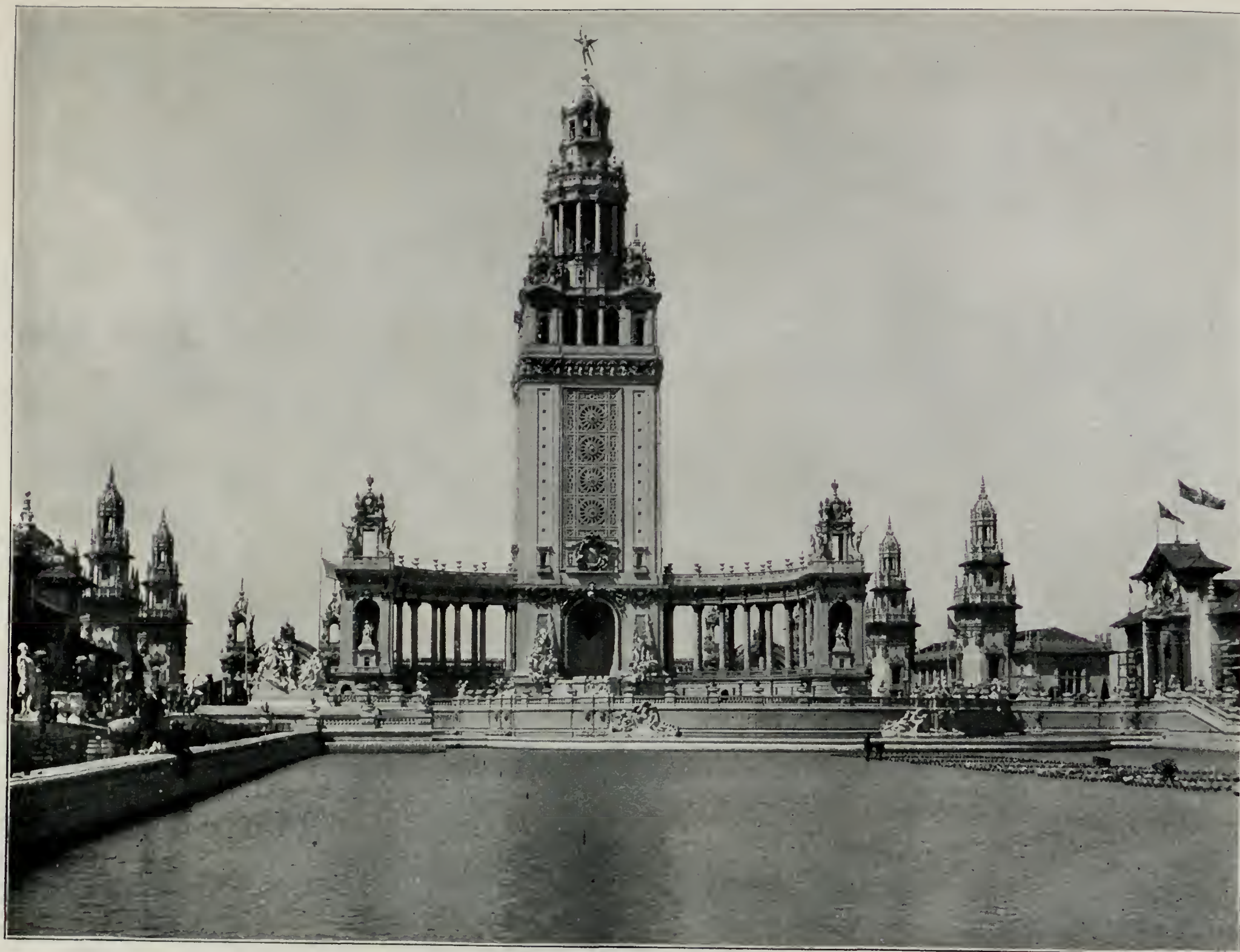
THE ELECTRIC TOWER
